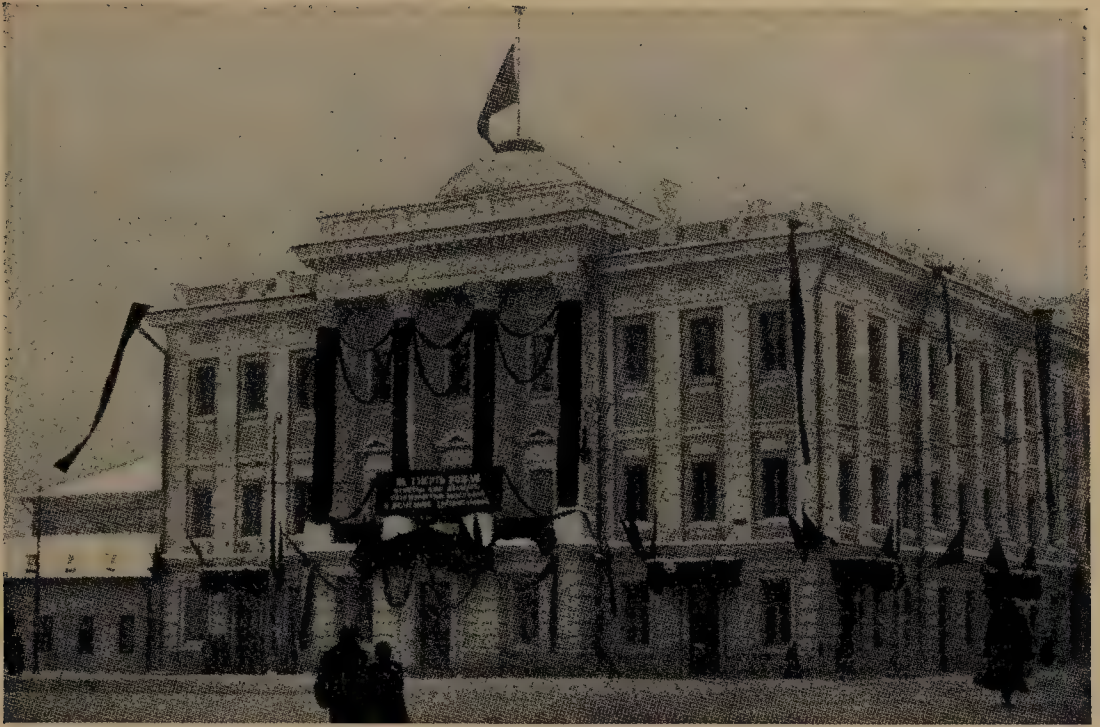
UNION BUILDING IN MOSCOW, IN WHICH LENIN'S BODY LAY IN STATE
